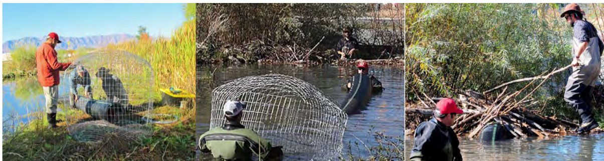
Figure 26: Pond leveler installation. From left: securing flexible pipe in cage to protect inflow from being clogged; placing pipe into beaver pond; rebuilding beaver dam after setting pipe into notched dam at desired water height.
